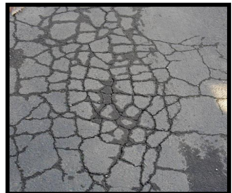
Figure 3.15.3c – Increased cracking
