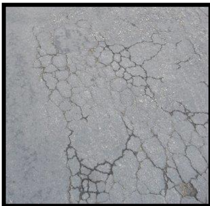
Figure 3.15.3b – Surface cracking
